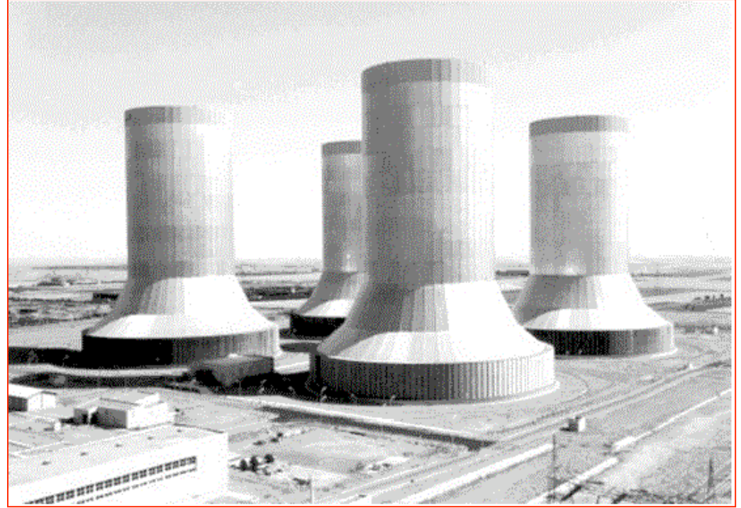
Earthquake Proof Natural Draft Towers for the Dry Cooling HELLER System of the 4 x 250 MWe Shahid Rajai PP (Iran)
